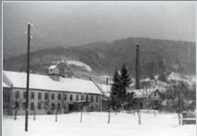
→ The backside of the factory on Albert-Hugard-Strasse, Staufen
